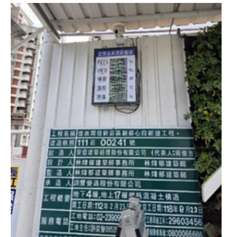
“Jiaxue.” Project: 5-in-1 Air Quality Information Display Panel
