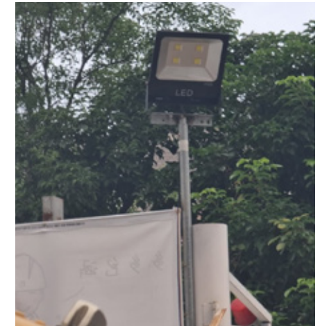
“Jiaxue.” Project Construction Site Fully Equipped with LED Lighting
